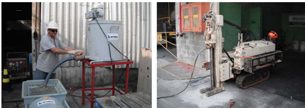
Figure 3. Preparation and direct injection of EHC-M slurry.
