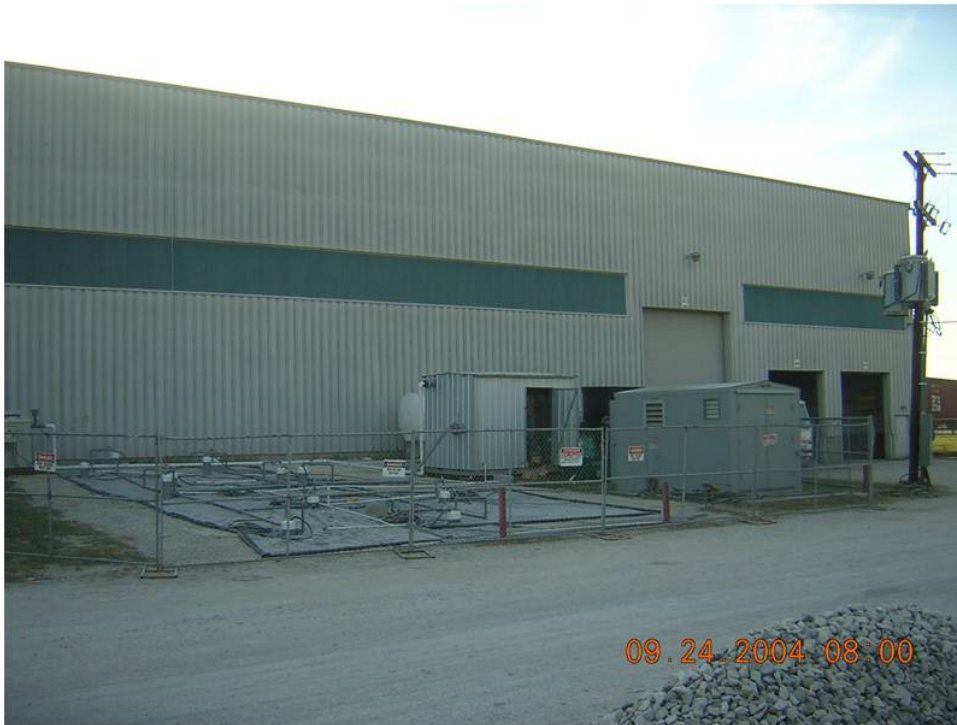
Figure 3. Site Photo with Equipment Compound
